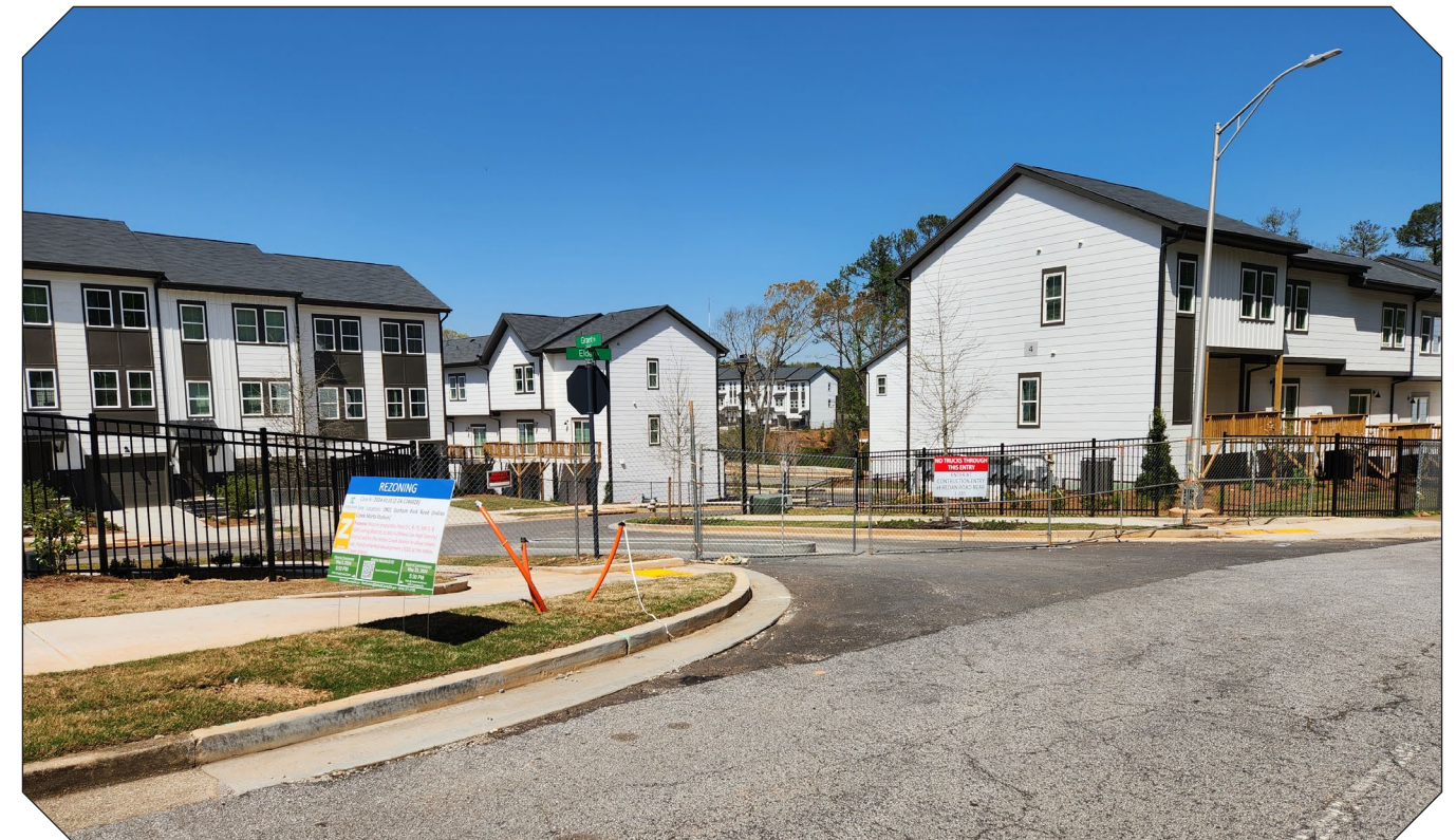
Generation Avondale east townhomes along Elder Lane.
