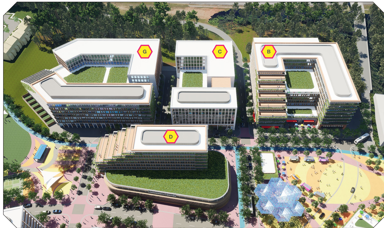
Blocks B, C, D, & G - Looking West
