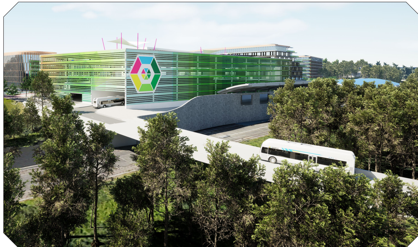
Phase 1A Parking Structure - Looking Southwest
