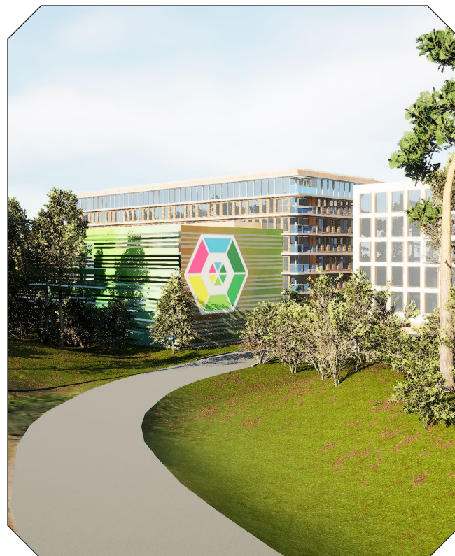
Block B Integrated Parking Structure - Looking Northwest from I-285 Off-Ramp
