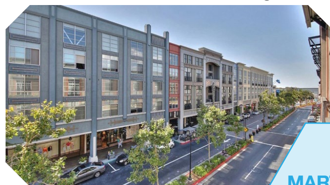
Station Area Development That Is Compact And Denser Relative To Its Surroundings
