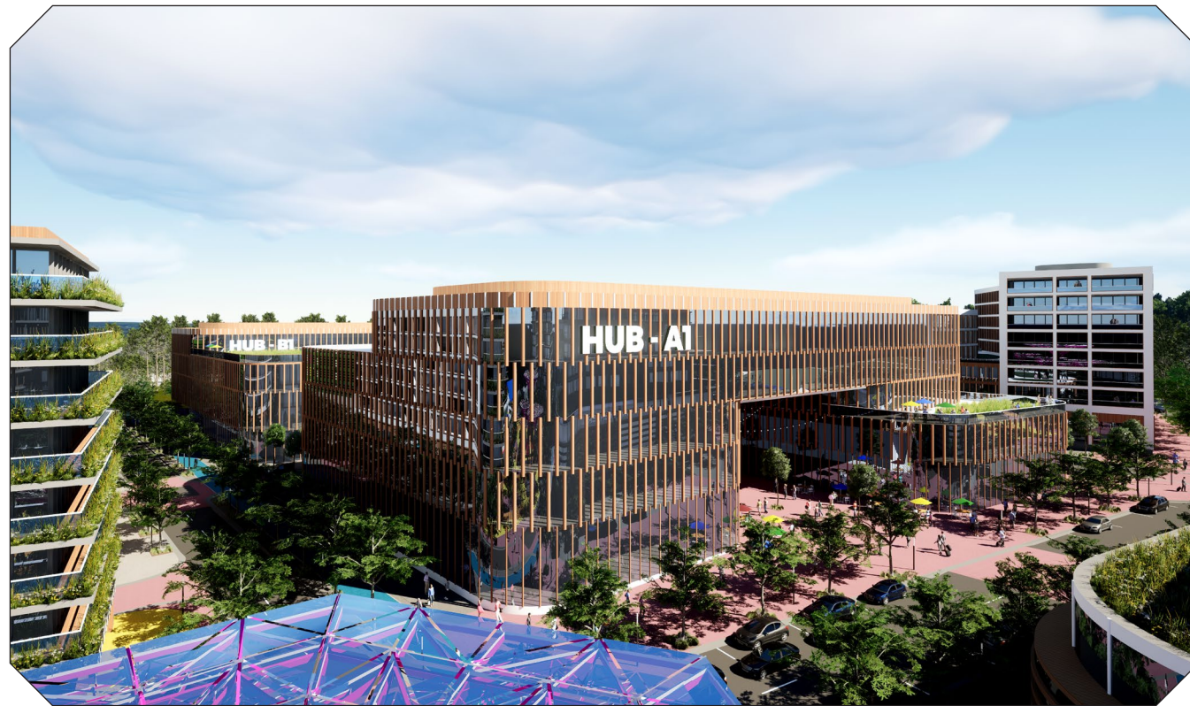
Hub A1 (Phase 4A) and Hub B1 (Phase 4B)
